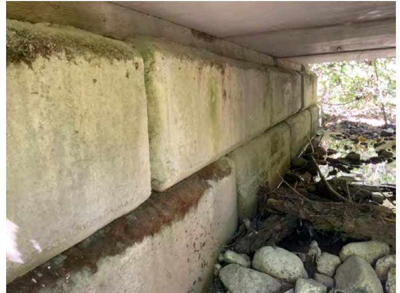
Right Bank Abutment when facing downstream
