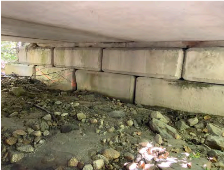
Left Bank Abutment when facing downstream
